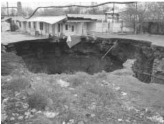
Fig. 1 Sinkhole above abandoned vertical shaft
