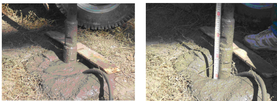
Figure 4. The situation of cement mortar before and after the discharge
