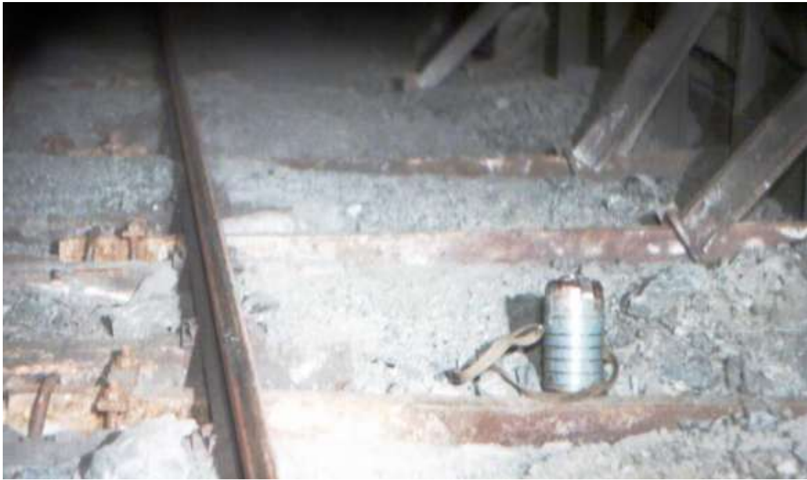
Figure 3 – Nature of look roadway floor with metallical cross floor bars and upright setting on belt entry of 7 th east longwall of a seam l_8^1 mine “Lidievka”
