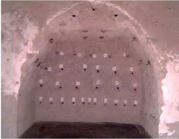
Fig. 4. A model of an excavation face with a curve-terrace form
