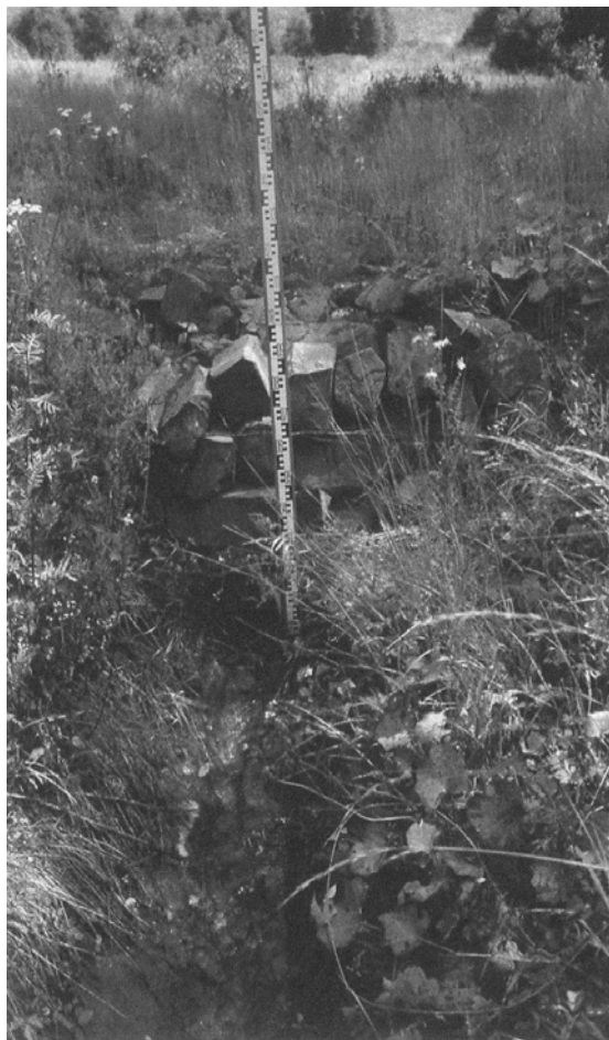
Fig.5. The motion of groundwater in the dump Fig.6. Rubble drain in the base of dump
